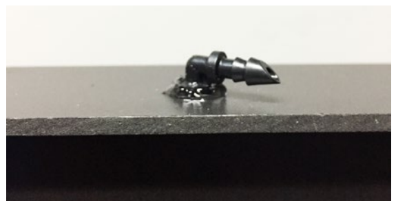
Installing an elbow
